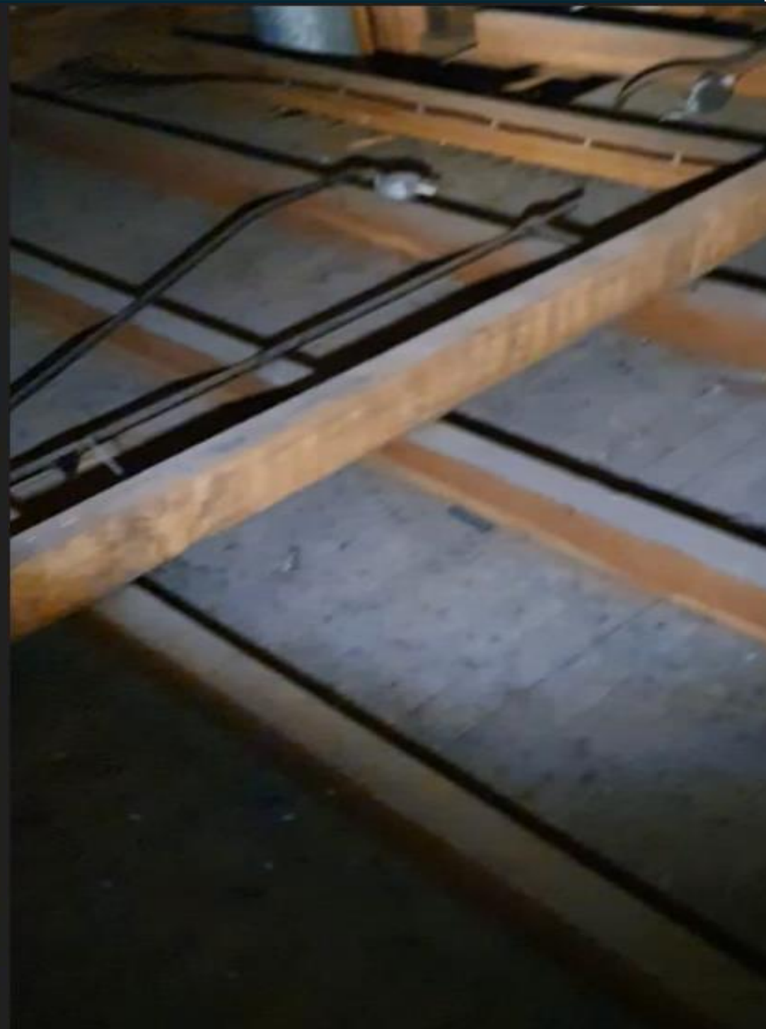
Current Insulation Situation in the Roof Space ( Currently there is No Insulation ) ( Example )
