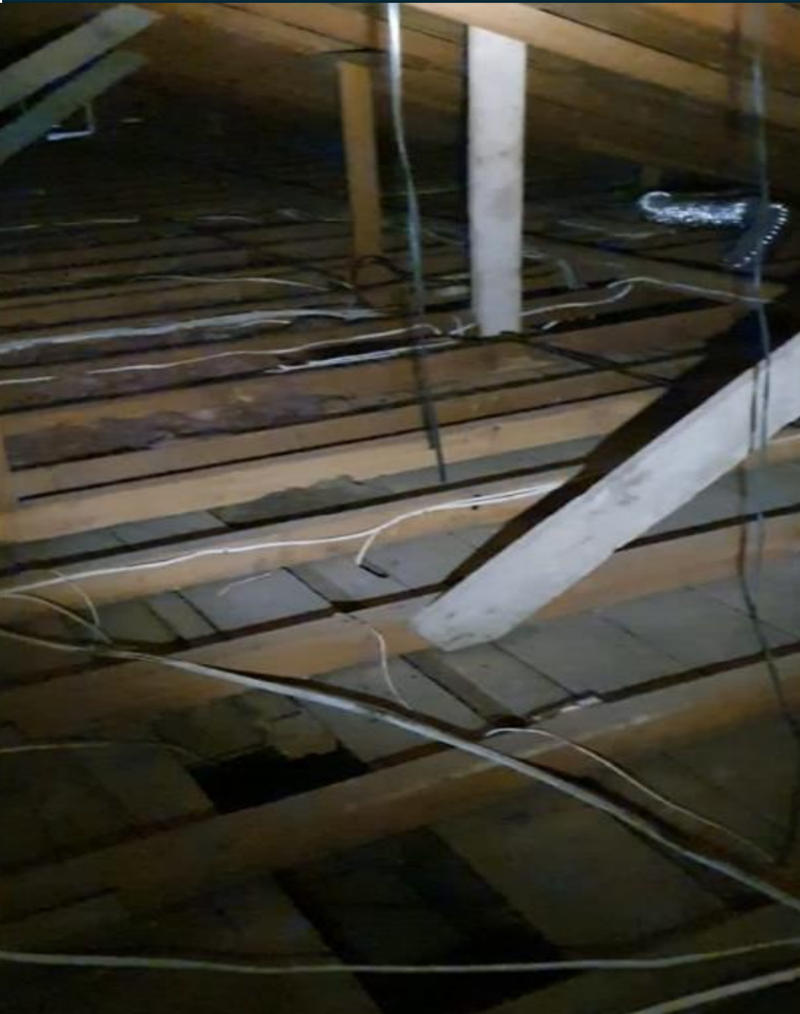
Current Insulation Situation in the Roof Space ( Currently there is No Insulation ) ( Example )
